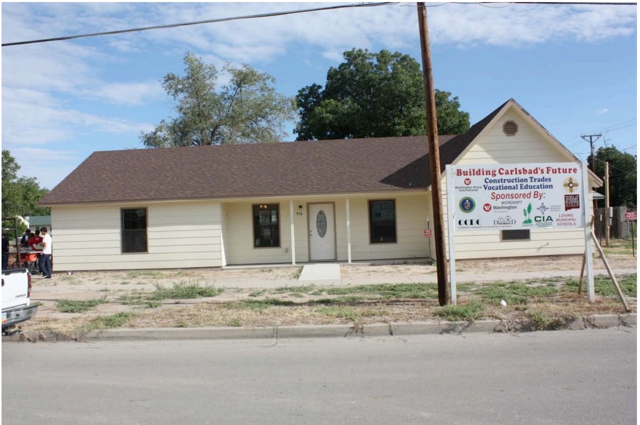
712/714 West McKay Street, Carlsbad, NM – CTVTP Third Home Build
