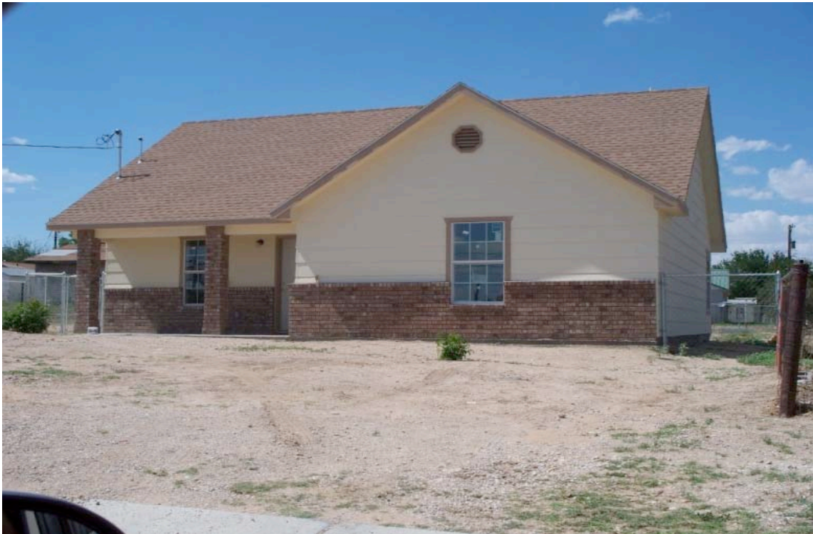
2512 West Wyoming Street, Carlsbad, NM – CTVTP Second Home Build
