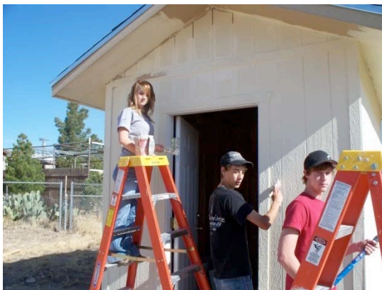
Wyoming Shed Build
